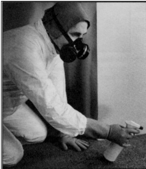
Mist carpet surfaces with water to reduce spread of dust.
